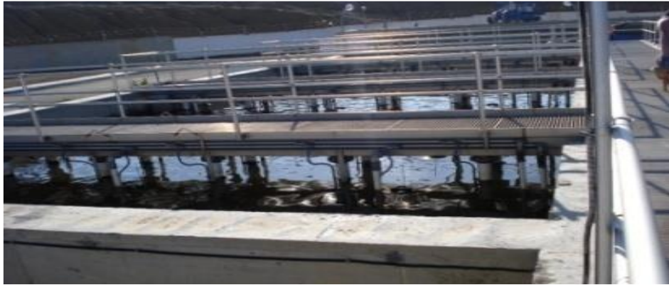
Figure III.5: Le clarificateur
