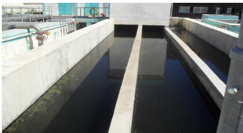
Figure III.7: Le bassin de chloration
