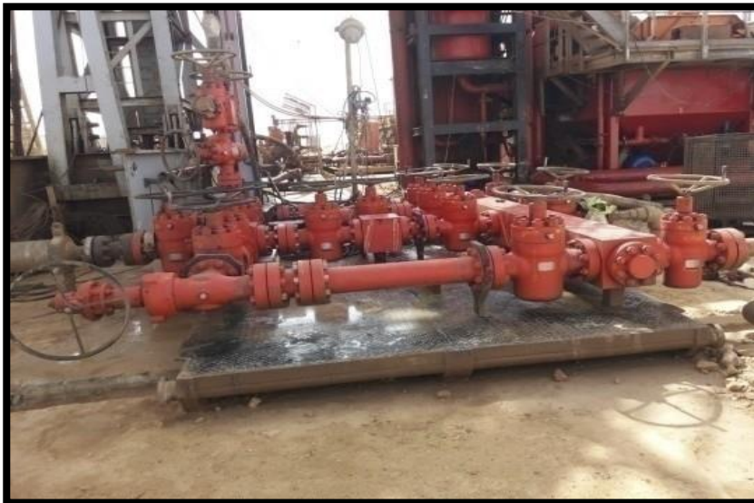
Figure II.6 : Chock manifold.
