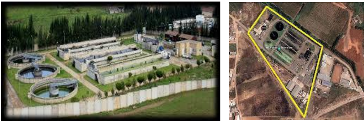
Figure 2: Station d'épuration Boumerdes
