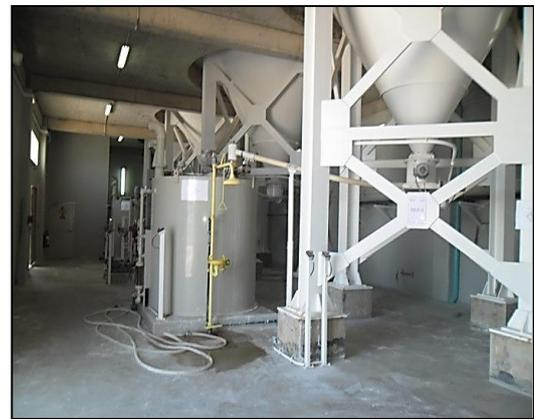
Figure III- 13: Silos de chaux
