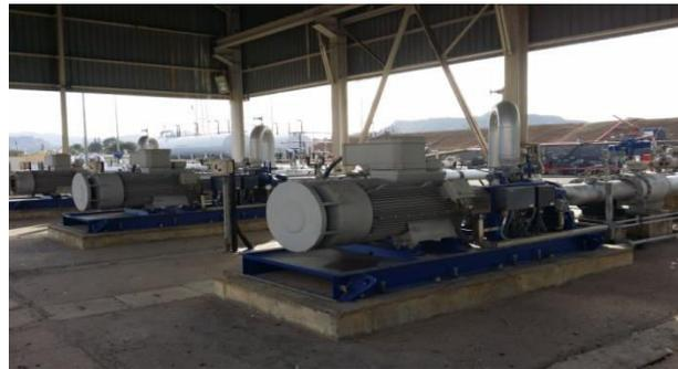
**Figure II.6 :** Pompes boosting.
