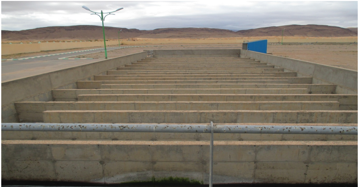
Figure III.10 : Bassin de chloration
