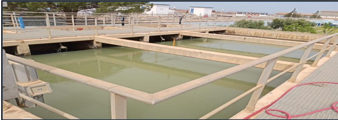
Figure II. 8: Photo chambre répartition
