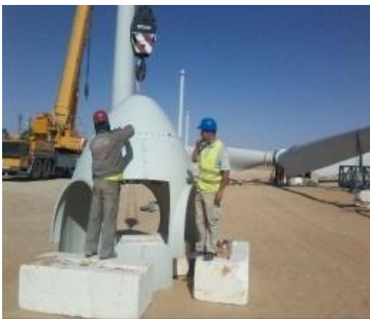
Figure IV.25 Montage de nose
