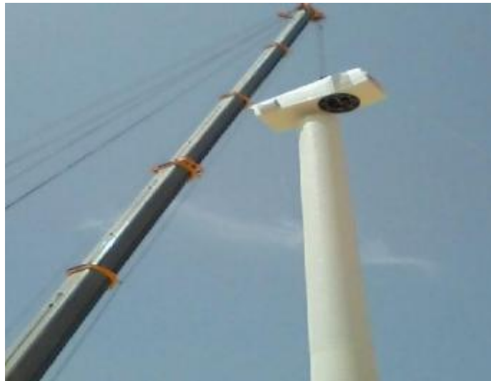
Figure IV.20 Levage nacelle
