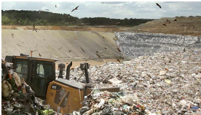
Figure I.7: Centre d'Enfouissement Technique (C.E.T).
