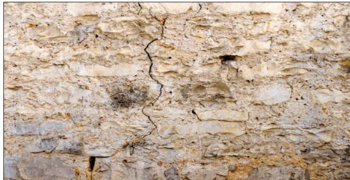
Figure I.27 : Fissures verticales
