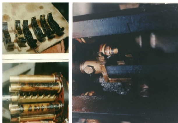
Fig. 3. Remove the particles by circulating the oil during the purification
