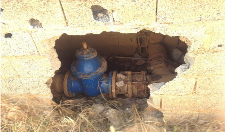
Figure III.1: robinet vanne
