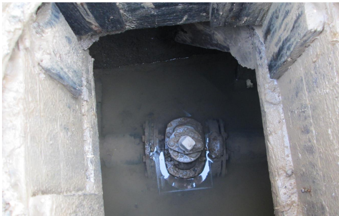
Figure IV.4: vanne opercule DN 150 PN16
