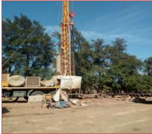
Figure 33: Installation de forage rotary en Djendel
