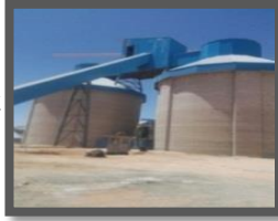
Figure II.12. Silos clinker SSC
