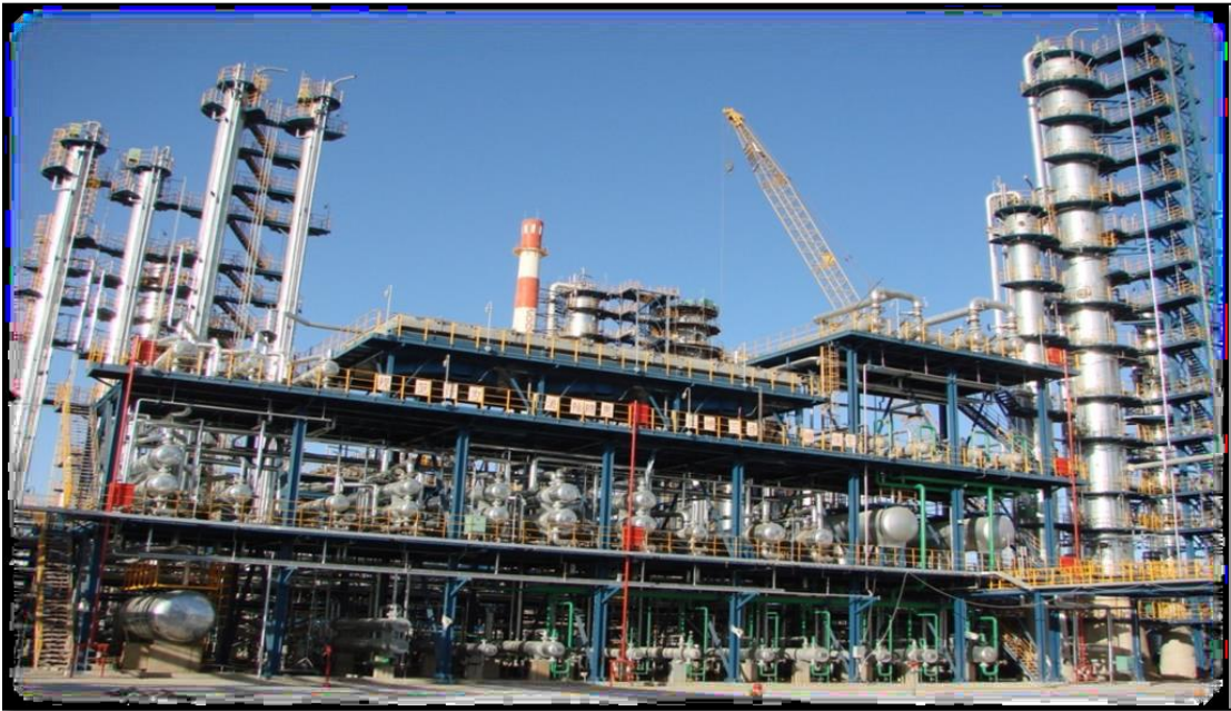
Figure I.3 : Unité CDU Topping.
