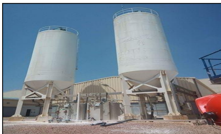
Figure III. 9: Silos de stockage de \text{CaCO}_3
