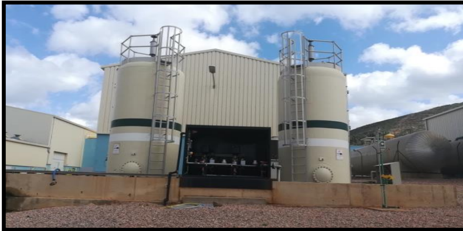
Figure 15: Usine de chloration
