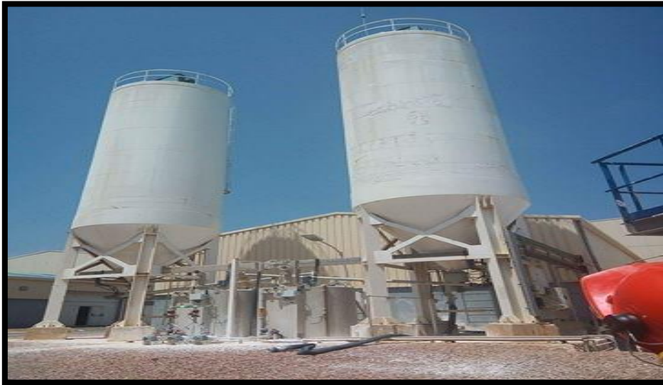
Figure 13: Silo de stockage
