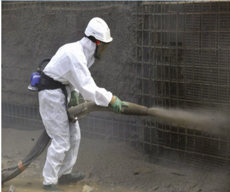
Figure [1.6] -béton projeté
