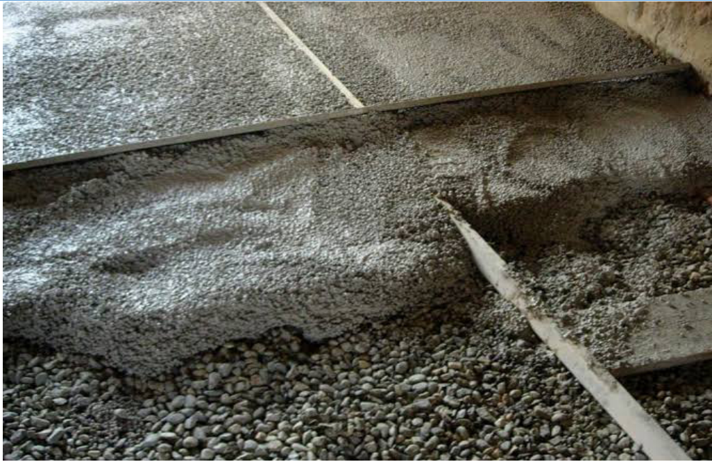
Figure [1.5] -béton léger
