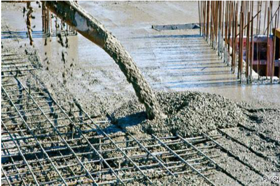
Figure [1.3] -béton armé
