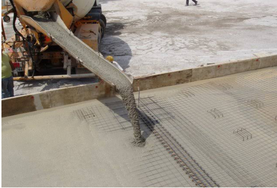
Figure [1.2] -béton auto plaçant
