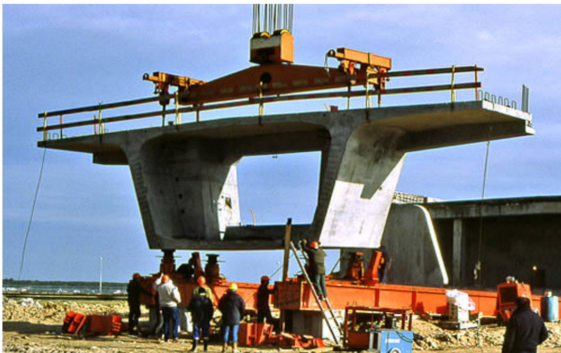
Figure [1.7] -béton précontrainte
