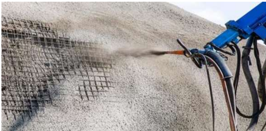
Figure III.6: Béton projeté.
