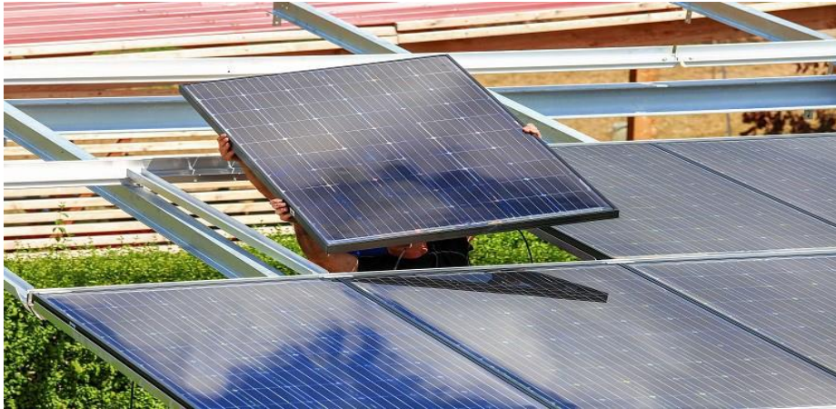
Figure 1-2 : Panneau solaire photovoltaïque [3]
