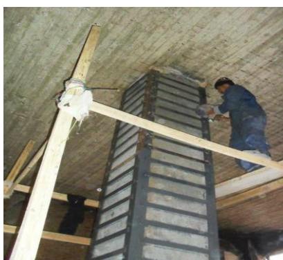
Figure II 23: Gainage métallique.
