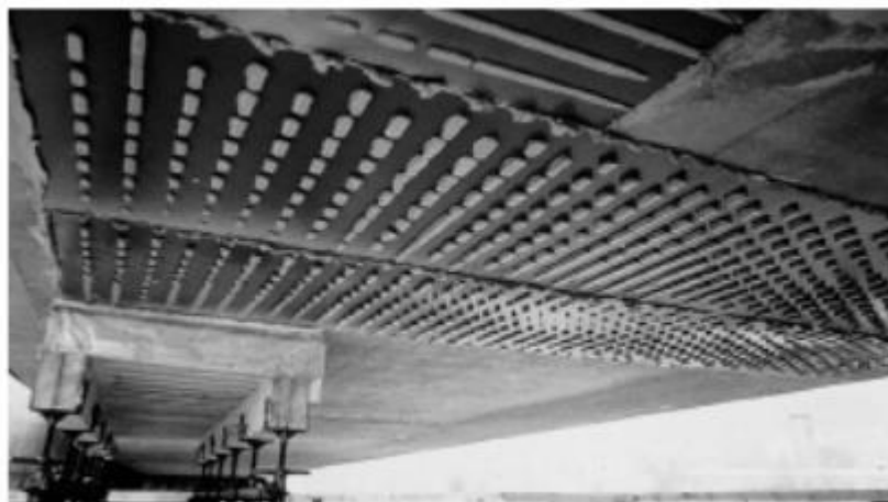
Figure II 20: Renforcement d'un viaduc.[5]
