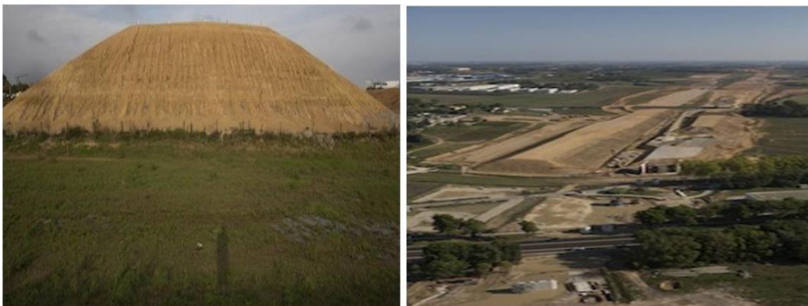
Figure 2: Exemples de Remblai
