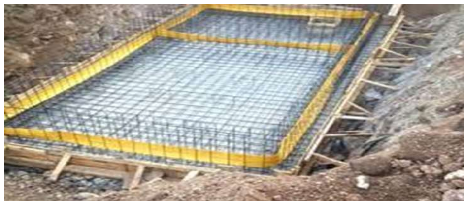
Figure I. 9 Water-stop
