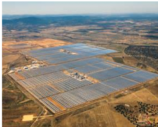
Figure (I .1): Centrale photovoltaïque.
