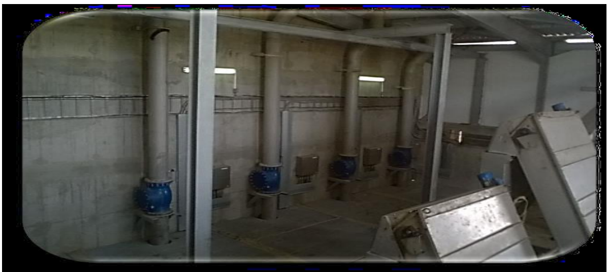
Figure 6: Les pompes de relevage
