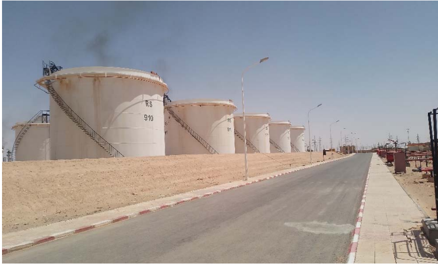
Figure II.1 : Bacs de stockage
