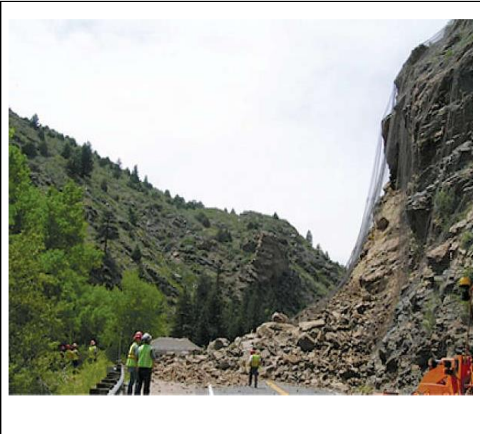
Figure I-6: A rockfall/slide that occurred in Clear Creek Canyon, Colorado, USA, 2005, [1]
