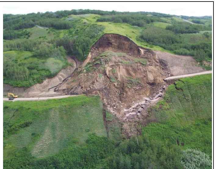
Figure I-12: A translational landslide that occurred in 2001 in the Beatton River Valley, British Columbia, Canada. [1]
