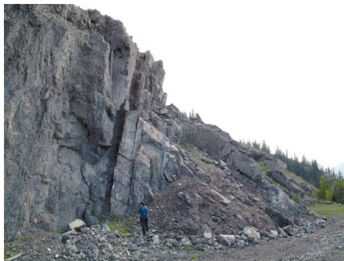
Figure I-8: Photography of block toppling at Fort St. John, British Columbia, Canada. [1]
