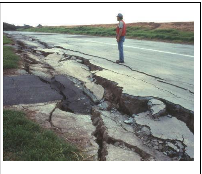
Figure I-14: Photography of lateral spread damage to a roadway as a result of the 1989 Lorna Prieta, California, USA, earthquake. [1]
