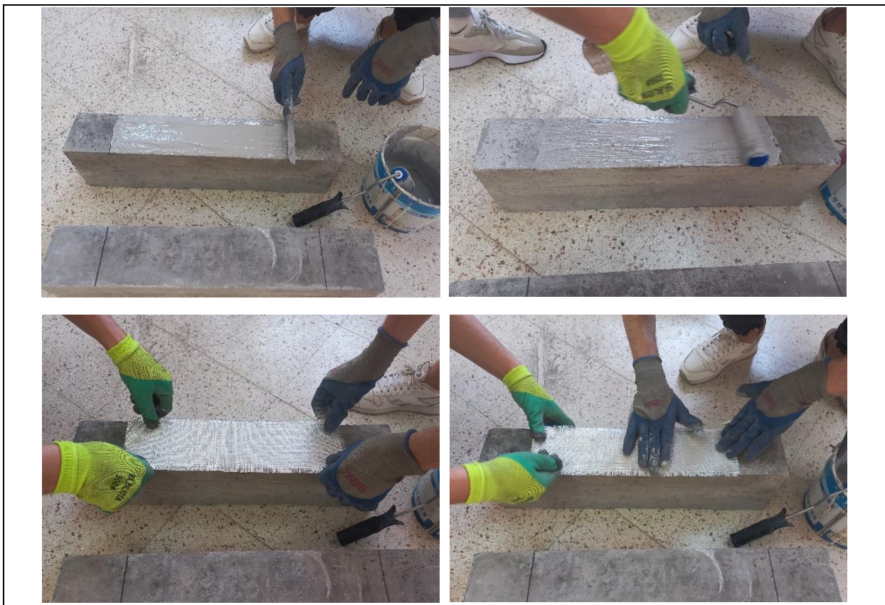
Figure III.12. Application du renfort
