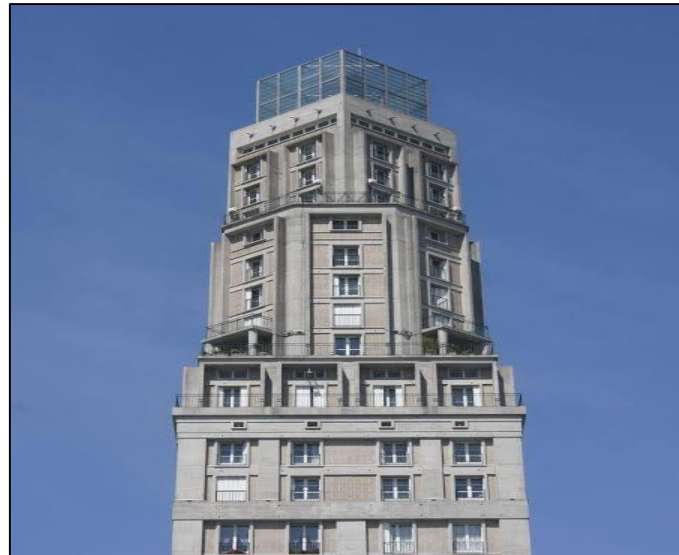
Figure I.2. La Tour Perret
