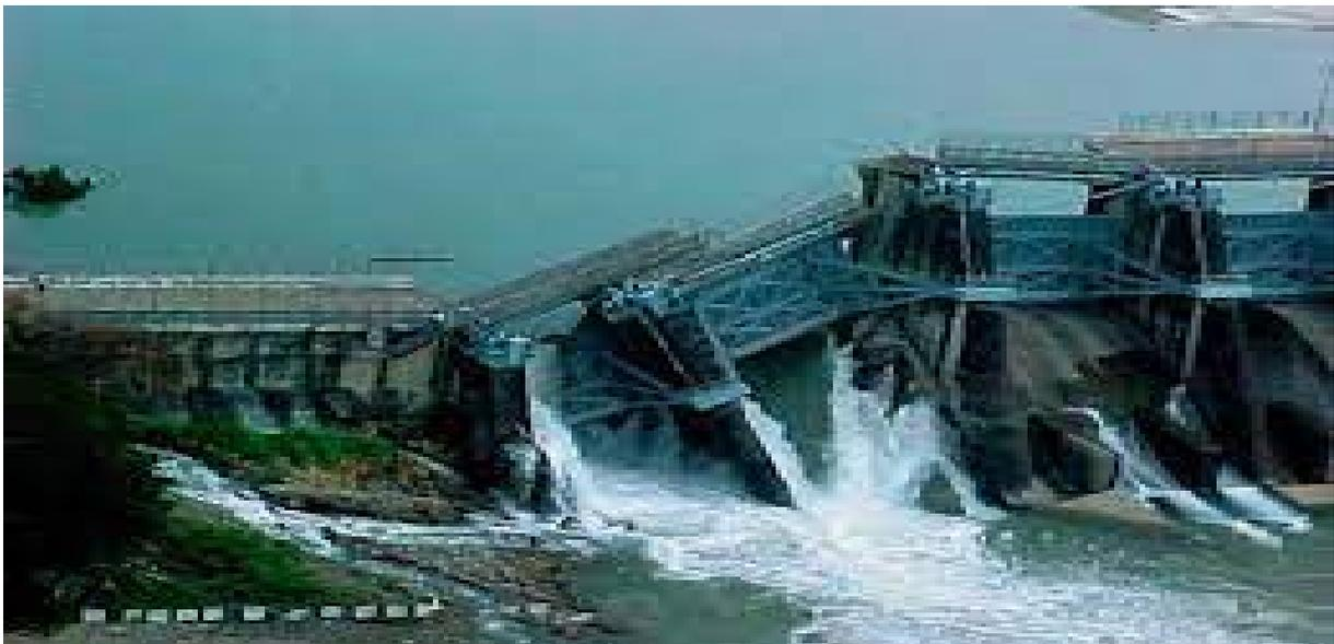
*Figure I.19: Rupture de barrage*
