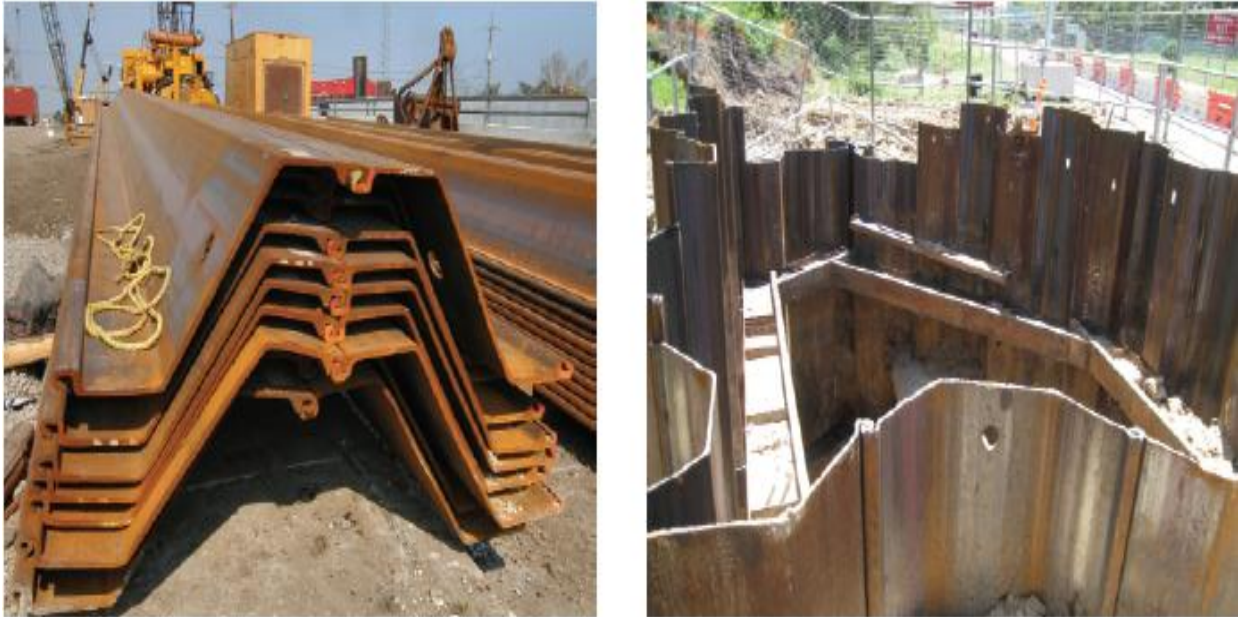
Figure I.11: Les rideaux de palplanches.
