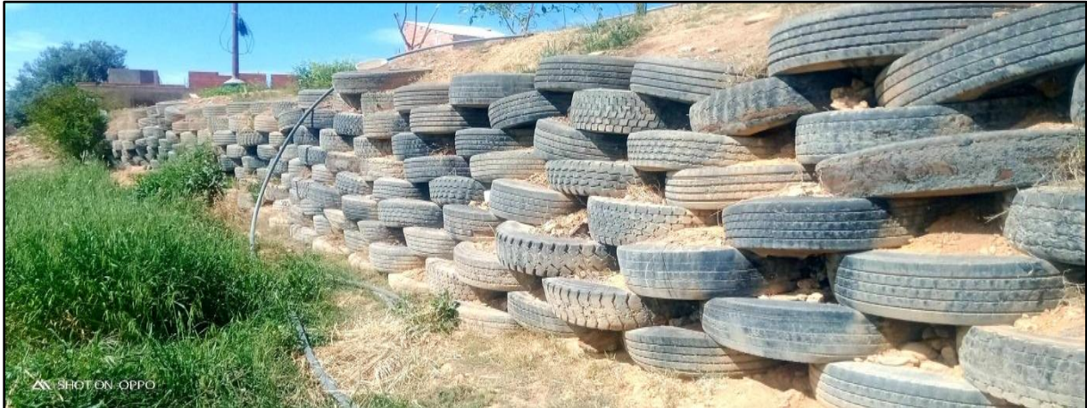
Figure I.6: Mur pneu sol (Bechloul).
