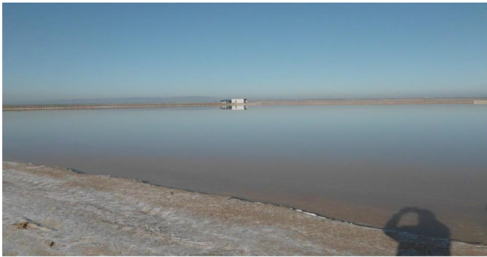
Figure 5: Station de pompage
