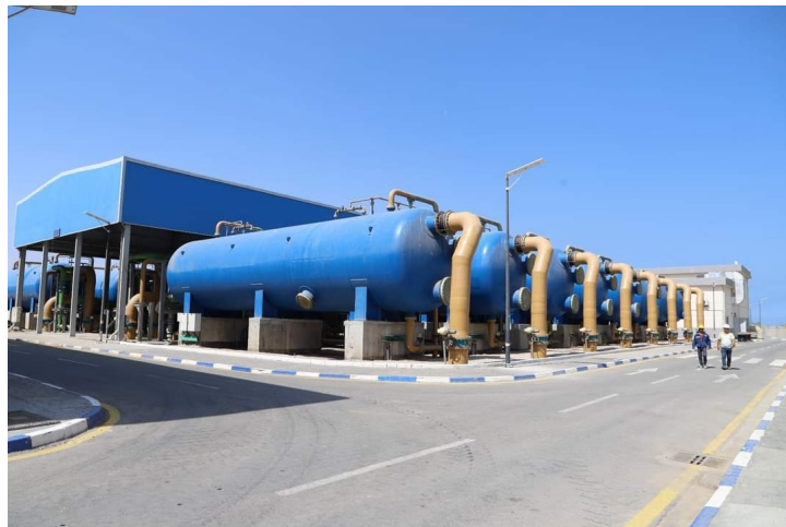
Figure III.9: Installation of sand filter
