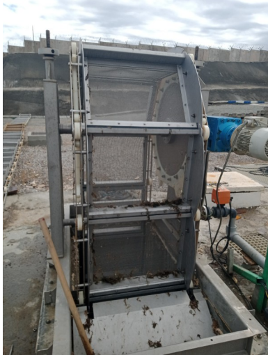
Figure III.7: The rotary screen
