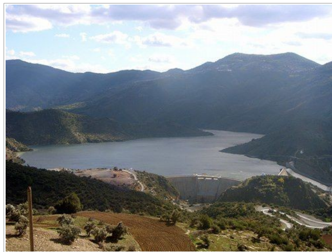
Figure II.1: Tichi Haf Dam [02]
