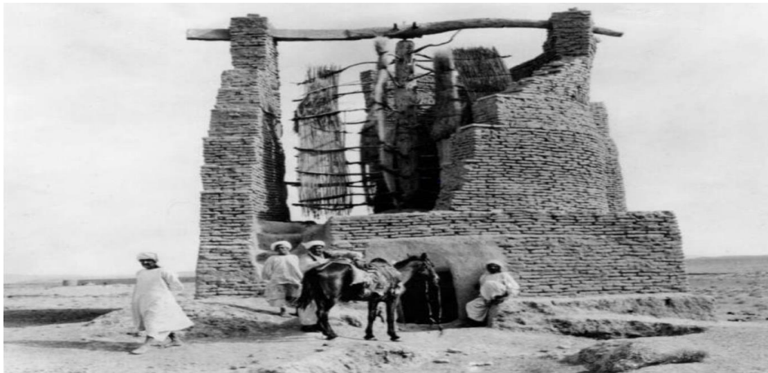
Figure 1.7 Vertical-Axis Windmill for Grain Milling, Afghanistan[8]
