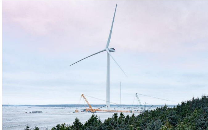
Figure 1.10 Vestas 33 V236-15.0 MW Large Scale HAWT [17]
