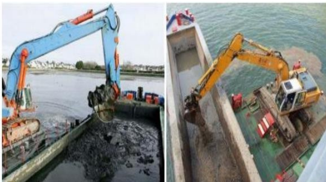
Figure II. 7: Dragage mécanique Dragage hydraulique
