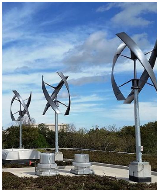
Fig. 1.5.VAWT generator structure.
