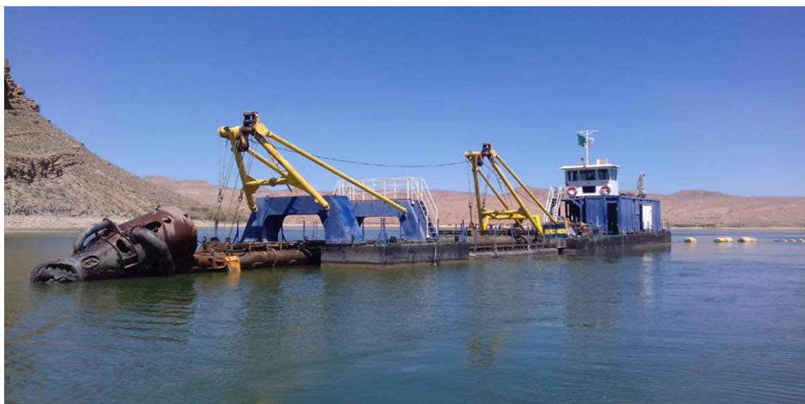
Figure III.10: Equipements drague du barrage K'sob M'sila (ANBT, 2016).
