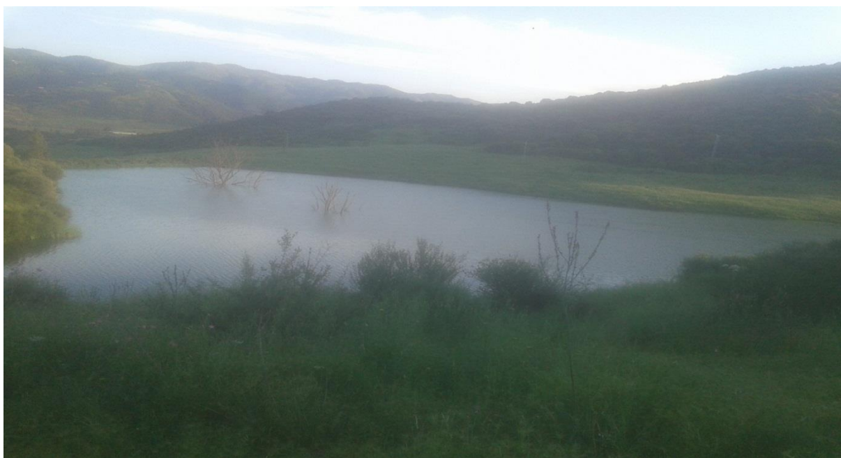
Figure III.6: Retenue collinaire à l'amont du barrage Beni Amrane (2018).
