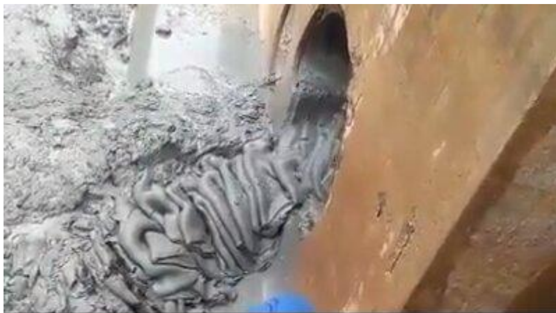
Figure III.8 : vidange de fond barrage k'sob (2018).
