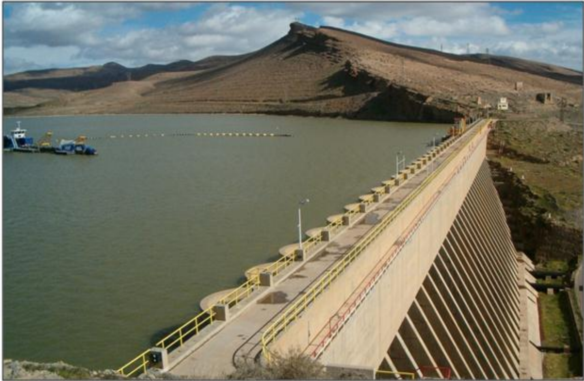
Figure IV.2 : Photo du barrage K'sob (2018).
