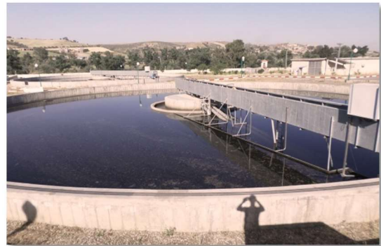
Figure 16 : Clarificateur (16/04/2017)
