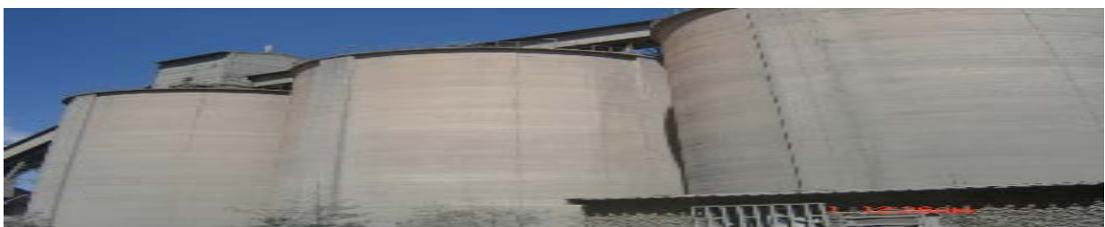
Figure II.11: Silos de stockage clinker
