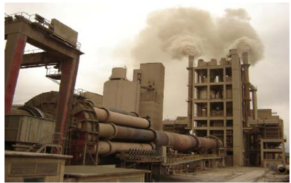
Figure II.10: Le four rotatif
