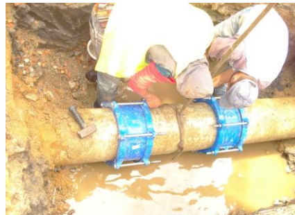
Figure 17:Manchon maxi (joint gibout)
