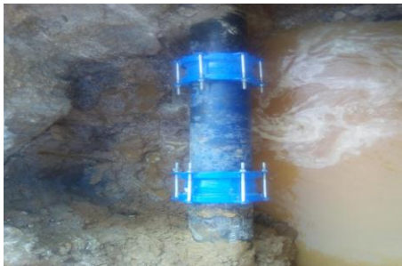
Figure 18: Manchon maxi joint gibault Conduite fonte Ø 200
