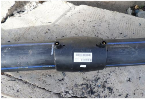
Figure16:Manchon a soudé
