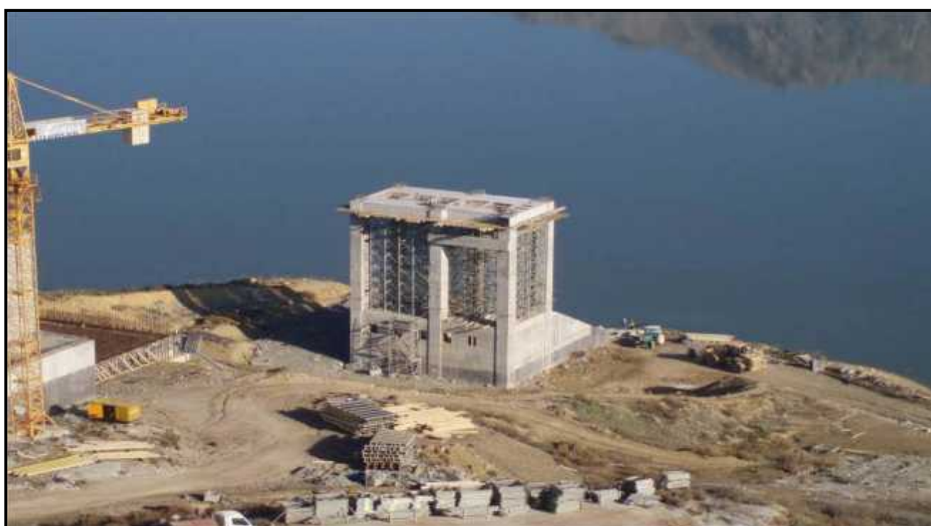
Figure 2 :L'exhaure (barrage Ighil-Emda commune Kherrata)
