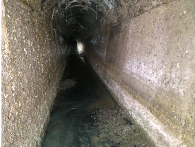
Figure N°6 : junction Dalot - ovoid (rue Med Bounafaa)/ovoid
