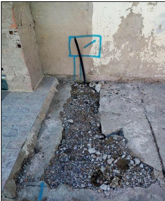
Figure V.7. Branchement (D=25mm)
