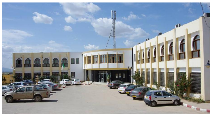
Figure I.1: ADWAN Chemicals Algeria
