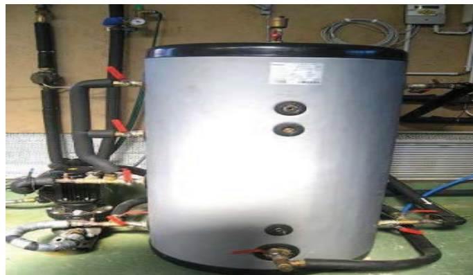
Figure (I.26) : Ballon de stockage chaud
