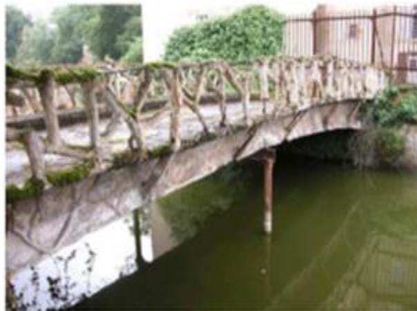
Figure II.2: Pont bi-poutre de Chazelet, 1875, Monier.
