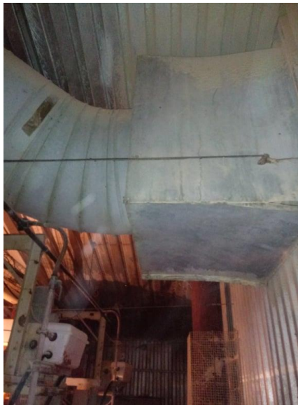
Figure 22: Source de chauffage (Photo personnelle, 2020).
