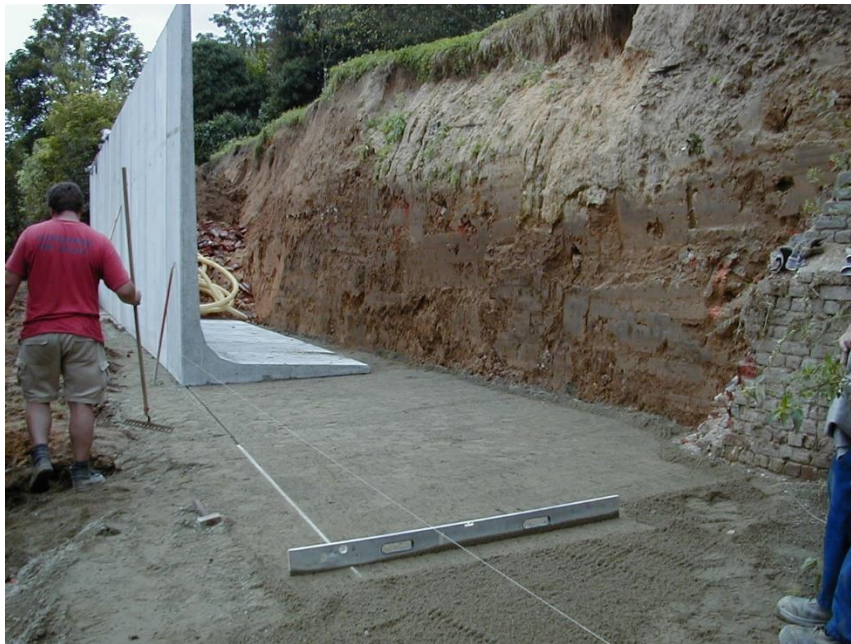
Figure I.4: Les murs cantilevers.
