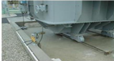
Figure 3.13: Placement de TC tore. .
